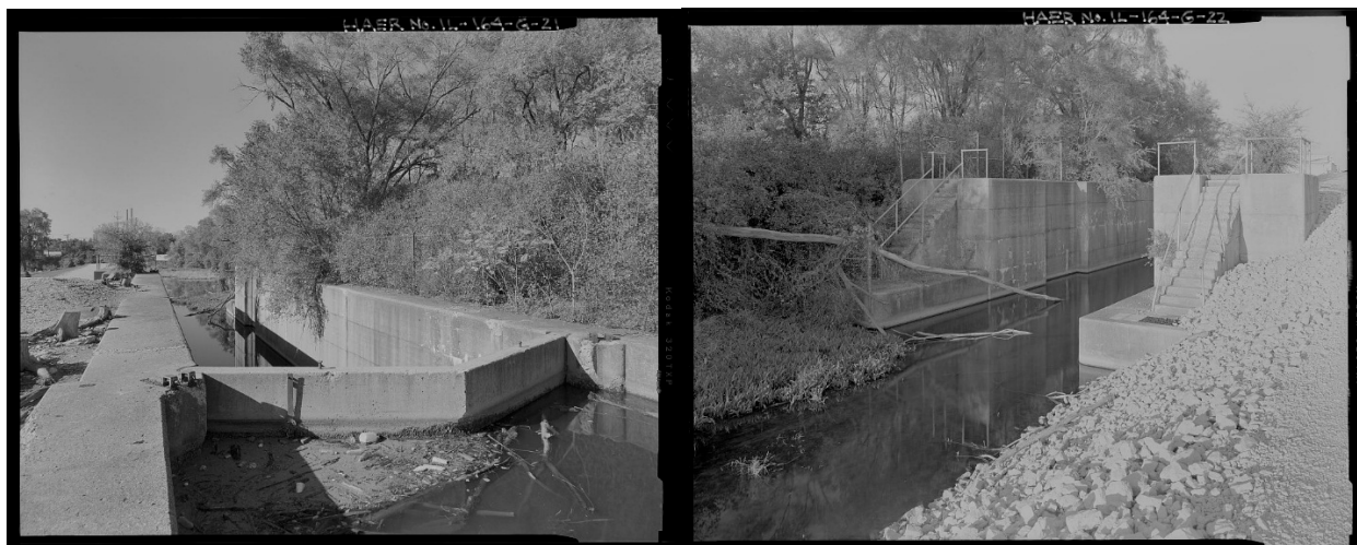
Figure 4-19 View of Remains of I&M Canal Lock Looking Downstream and Upstream, Respectively (Source: Christianson 2008)
