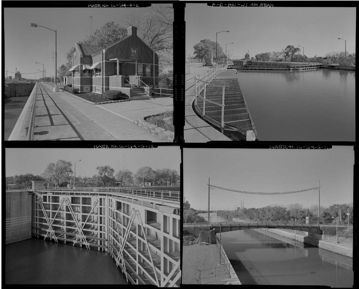
Figure 4-18 View (from top left to bottom right) of Control Station and Lock Looking Southwest; View of Upstream Lock Gate in Closed Position and Auxiliary Gate in Open Position; View of Exterior Detail of Downstream Lock Gates Looking Northwest; and View of Brandon Road Bridge from Downstream Lock Gate Looking South Southwest (Source: Christianson 2008)
