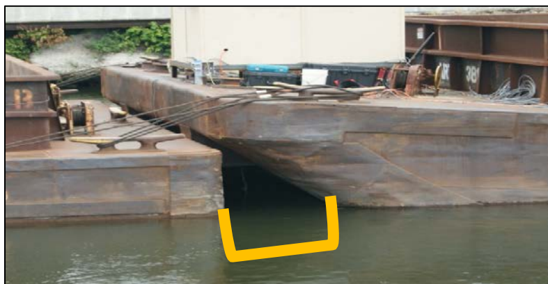
Figure 6-6 Spaces between Barges Where Fish and Floating ANS May Be Entrained
