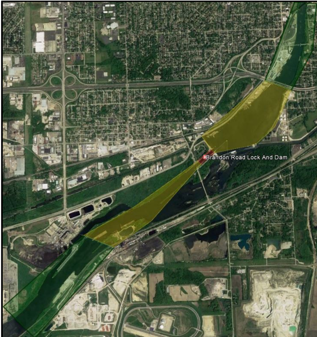
Figure 4-20 Aerial View of BRLD (Yellow polygons indicate the arrival area for vessels wishing to utilize the lock chamber and represent where processing time begins. The red polygon identifies BRLD; movement through the lock and dam is also included in processing time.)
