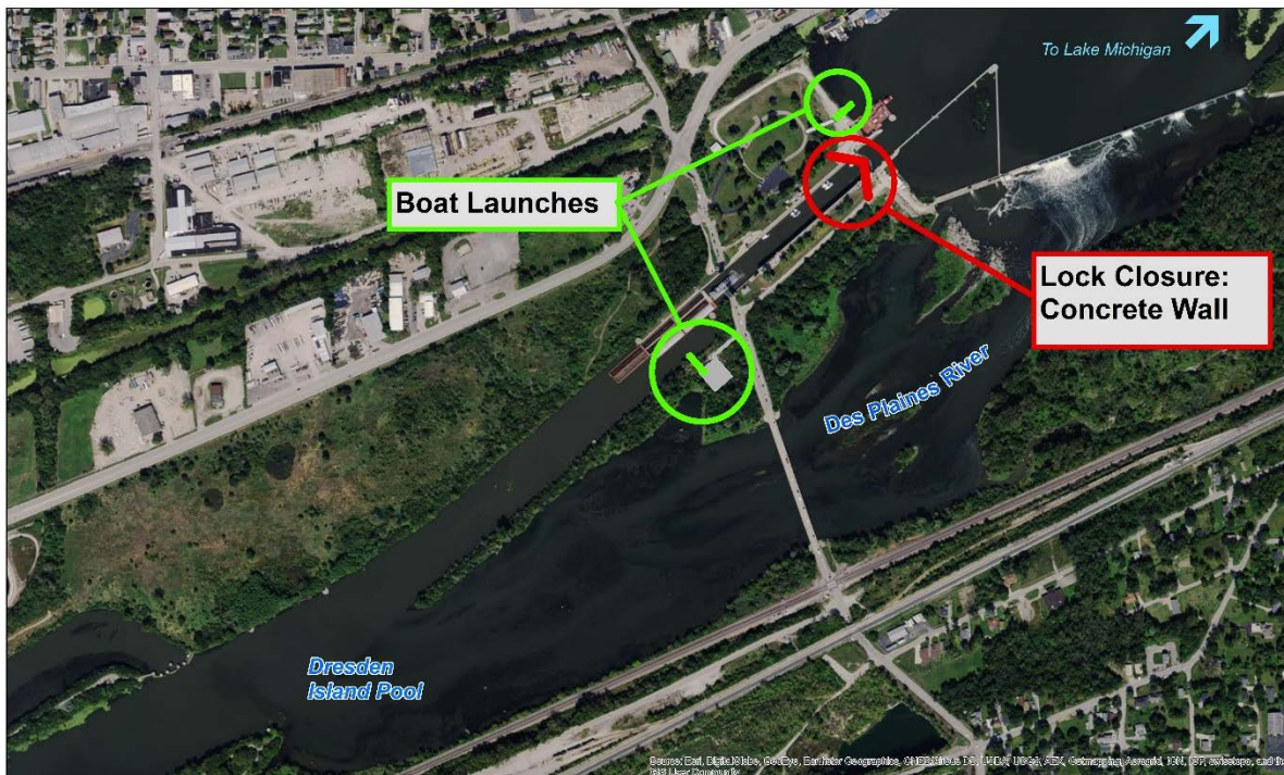
Figure 6-43 Aerial View of BRLD with Potential Layout of Lock Closure Alternative
