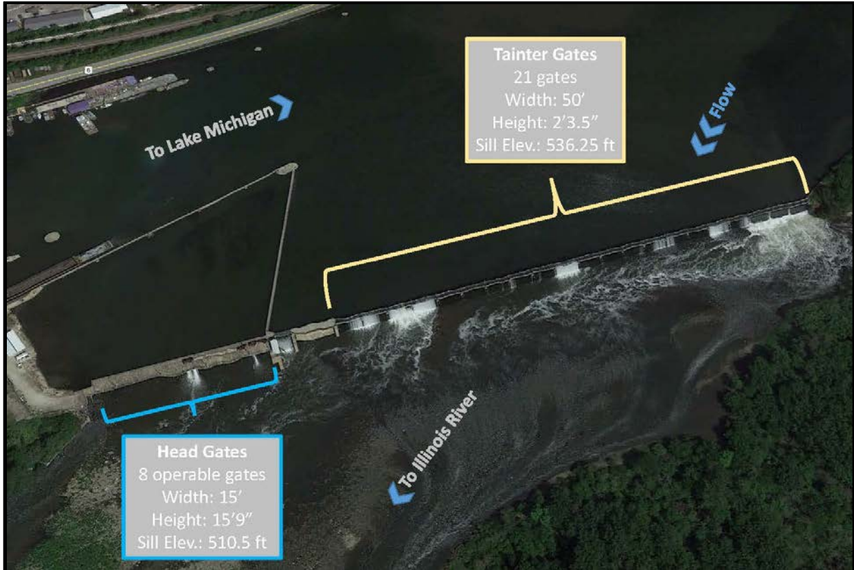
Figure 1-7 BRLD Aerial View Showing Head Gate and Tainter Gate Characteristic
