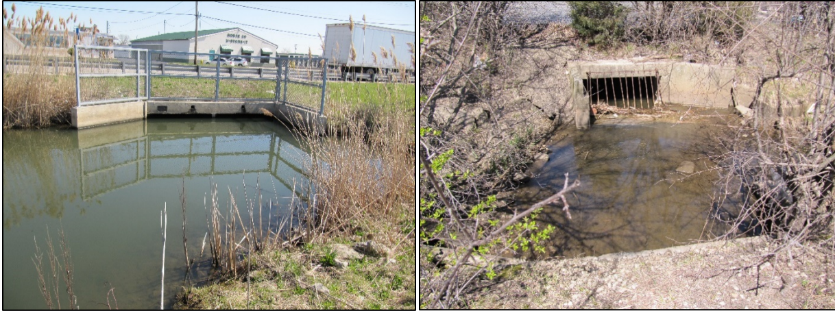
Figure 6-19 Left: Downstream End of the Box Culvert That Travels Approximately 0.10 mi (0.2 km) under Plainfield Road and Several Parking Lots and Buildings; Right: Upstream End of the Culvert, Which Has a Trash Rack on the Entrance with 4 to 6 in. (10.2 to 15.2 cm) Gaps between the Rebar
